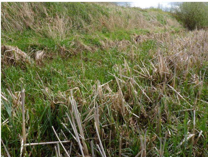
Photograph 9. Ditch channel overgrown with monocots (view to S)
