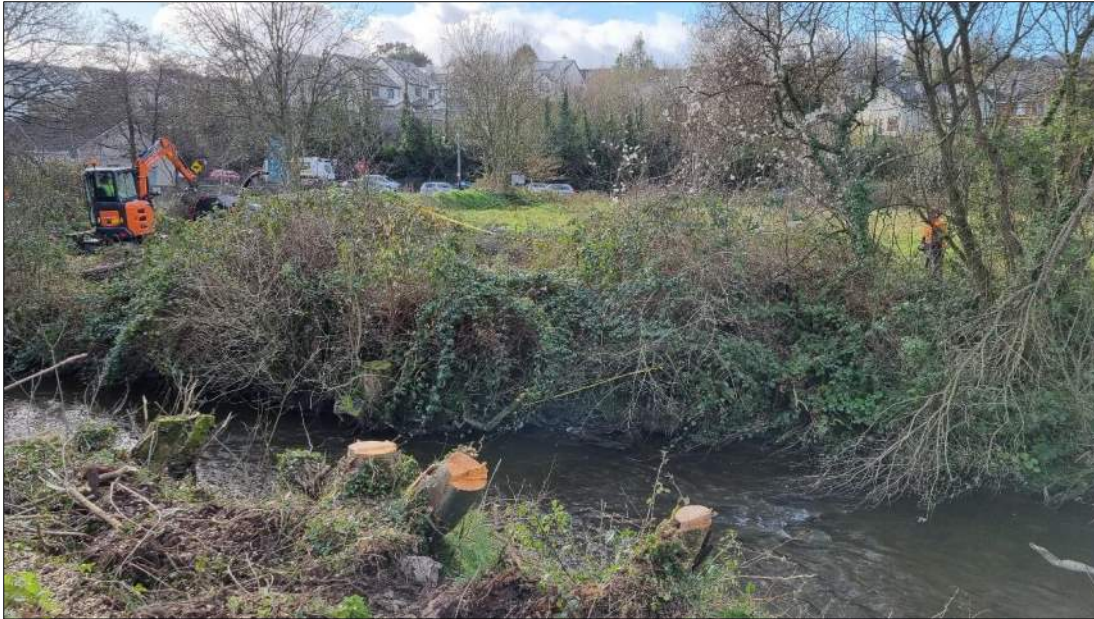
Plate 3.1 Tree felling in the 'Circus Field' at Meadowbrook showing the preservation of vegetation overhanging holt No. N6 on the Glashaboy River at Meadowbrook. Vegetation area that was preserved overhanging the holt was marked with yellow hazard tape from above to ensure drivers avoided inadvertent cutting
