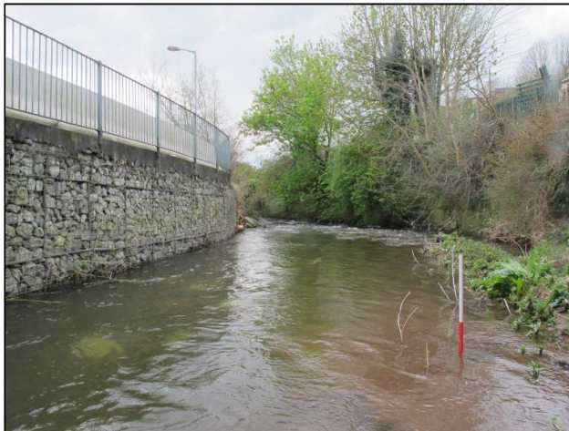
Plate 107: South-facing view of river channel on the upstream side of Orchard Court (1m scale).
