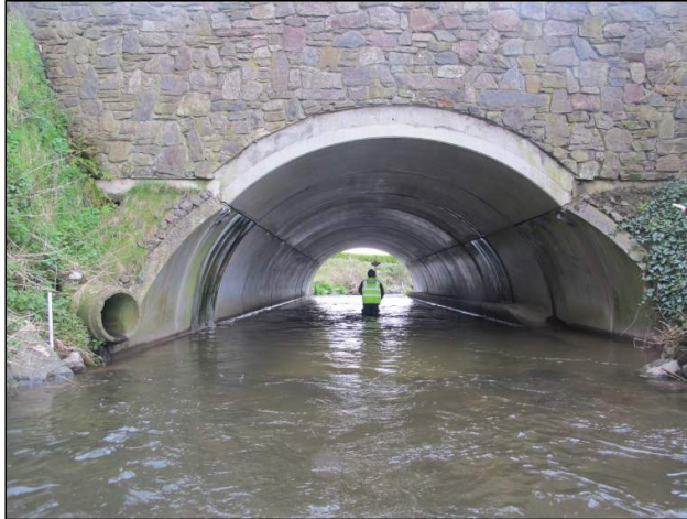
Plate 97: Upstream side of concrete culvert that accommodates a road bridge on the downstream side of the parkland area (1m scale).
