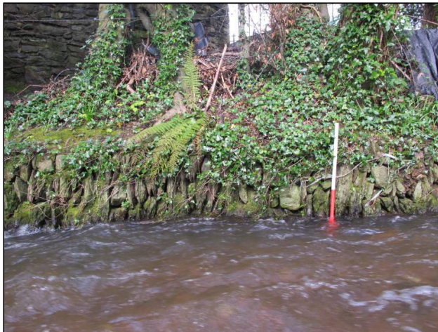
Plate 149: River-walling (Feature F08) located downstream of bridge (Feature F07) at entrance to Kilnap Glen House (1m scale).
