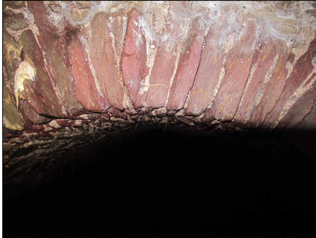
Plate 169: North-facing view of section of arch-ring from culvert, Feature F14B, which abuts culvert Feature F14A.
