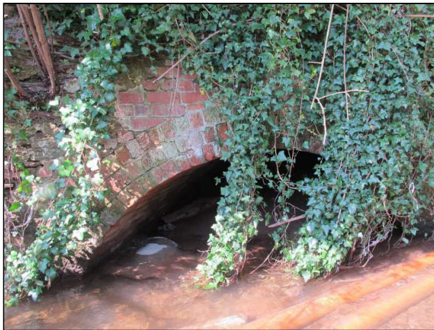
Plate 122: Modern, brick-built, culvert that drains into the river channel on its west side.
