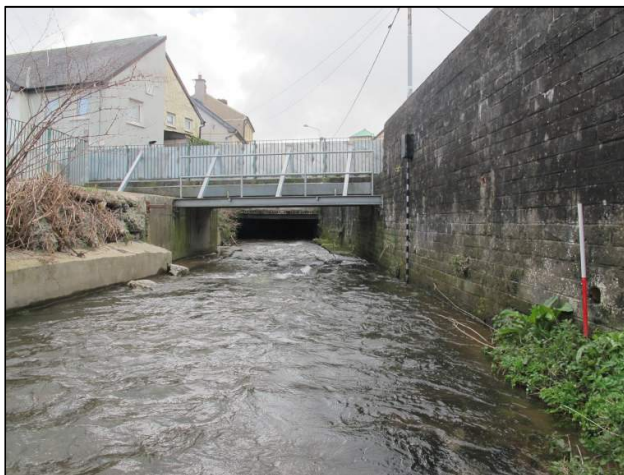
Plate 114: South-facing view of river channel upstream from sedan pedestrian access bridge. Note entrance to 68m-long modern culvert in distance (1m scale).
