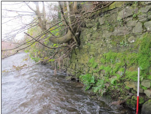
Plate 155: River-walling (Feature F10) located along west side of river channel at Orchard Court (1m scale).
