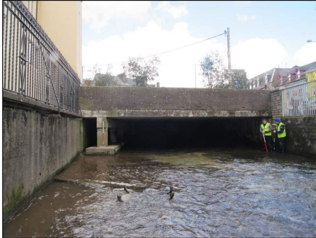
Plate 115: North-facing view of downstream side of 68m-long section of modern culvert running between Blackpool Bridge and the Church of the annunciation.
