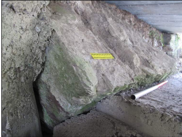
Plate 160: Detail shot of springing arch-stone from base of the removed arch at Feature F11 (15cm/ 1m scales).
