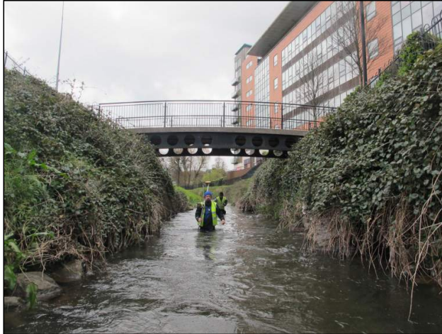
Plate 94: View of river on downstream side of a second footbridge that crosses the channel within the parkland area.
