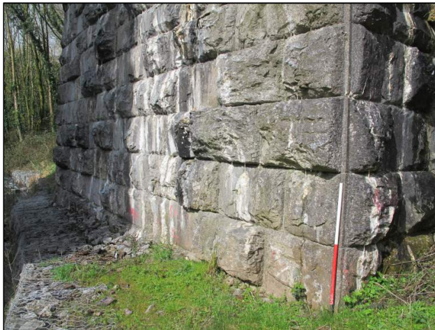
Plate 134: Southwest-facing view of the arch-wall on the western side of Arch No. 4 (1m scale); note use of rock-faced masonry.
