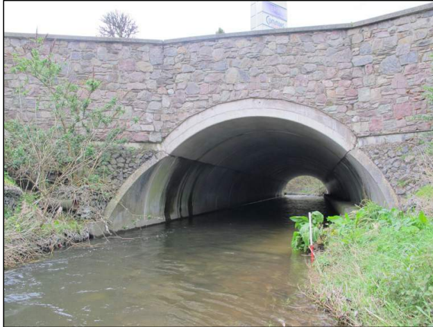
Plate 100: Upstream view of modern culvert that accommodates river-flow beneath the N20 roadway (1m scale).
