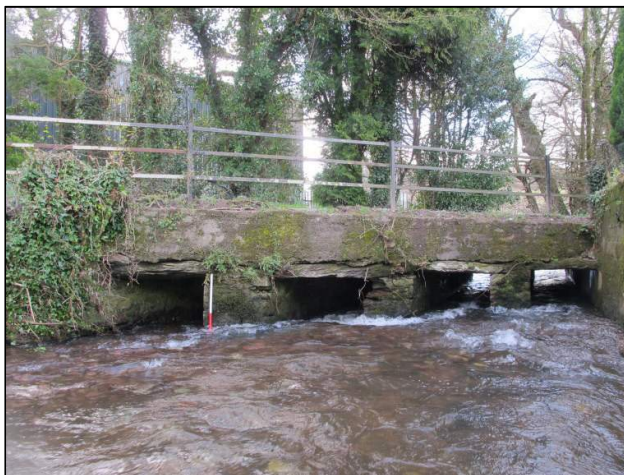
Plate 144: South-facing view of upstream side of a 'clapper' style bridge (Feature F07) at entrance to Kilnap Glen House (1m scale).
