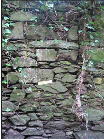
Plate 172: Example shot showing composition of river-walling comprising Feature F15B (15cm scale).
