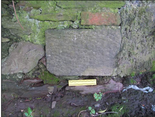
Plate 157: Detail shot of piece of well-dressed masonry (CS17) re-used in construction of river-walling, Feature F10 (15cm scale).
