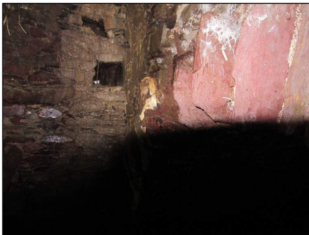
Plate 168: Internal shot showing point at which Feature 14A abuts another masonry culvert, Feature 14B; see Figure 19 for location.
