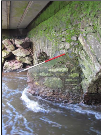
Plate 152: North-facing view of triangular cutwater on upstream side of masonry bridge (Feature F09) at Fitz's Boreen (1m scale).
