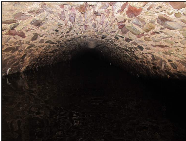
Plate 170: Internal shot of Intrados from section of culvert, Feature F14B.
