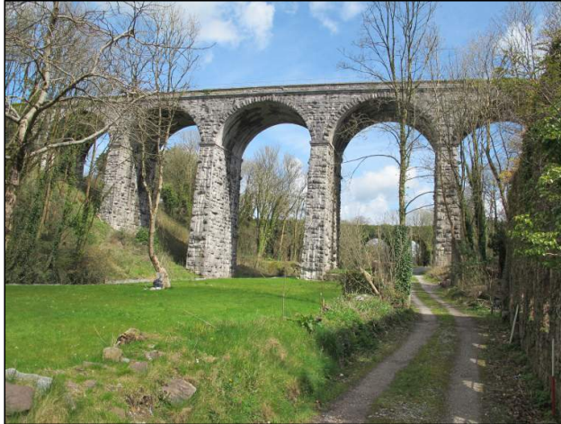
Plate 133: Northeast-facing view of the downstream side of Kilnap Viaduct, Feature F03 (1m scale).
