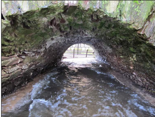
Plate 154: Internal view along Arch No. 2 from masonry bridge (Feature F09) at Fitz's Boreen.
