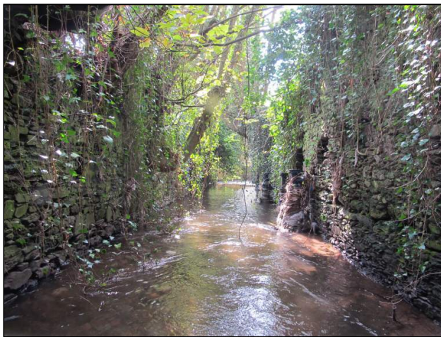
Plate 171: South-facing view of river channel with high sections of opposing river-walling (Features F15A and F15B).
