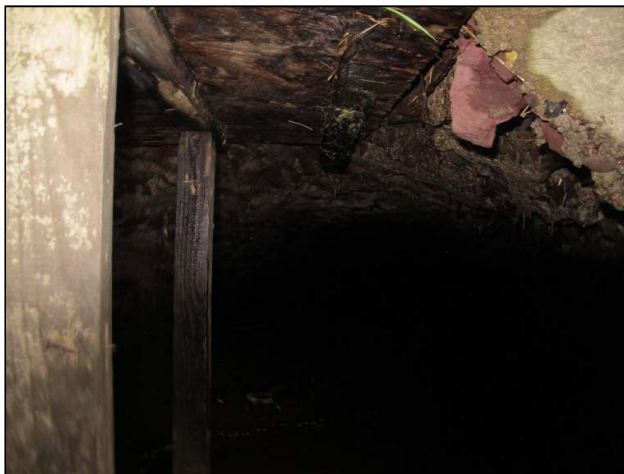
Plate 165: Internal shot showing masonry culvert (Feature F13) located behind a modern culvert opening.
