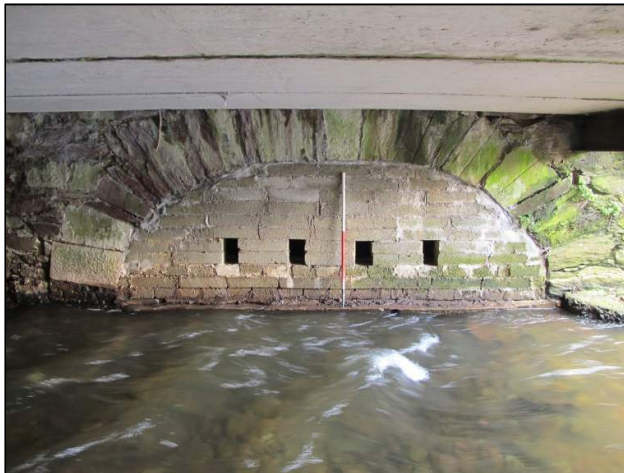
Plate 161: Masonry culvert arch (Feature F12) located beneath modern culvert (1m scale); see Figure 18 for location.
