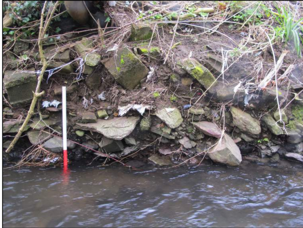
Plate 103: East-facing example view of the composition of the eastern bank structure (1m scale).
