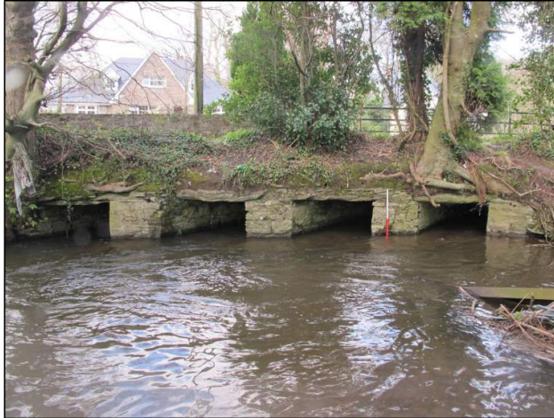
Plate 145: North-facing view of downstream side of 'clapper' style bridge, Feature F07 (1m scale).
