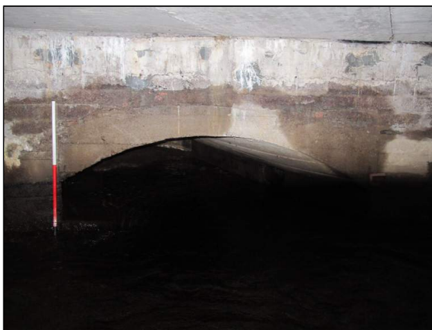
Plate 117: Small (modern) culvert that drains into the river, on its east side, within the larger culvert (1m scale).
