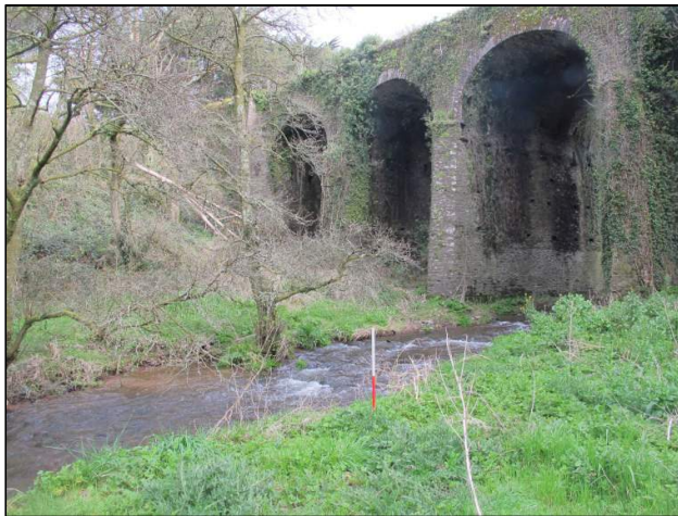
Plate 125: North-facing view of downstream side of Kilnap Bridge (Feature F01).
