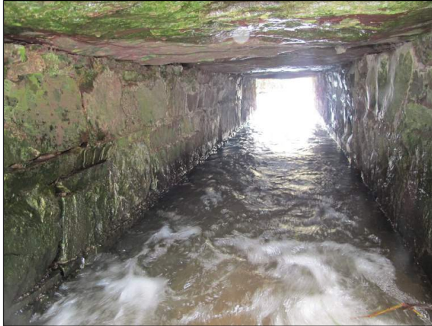
Plate 148: Internal view of pier walls and ceiling stones from 'clapper' style bridge, Feature F07.
