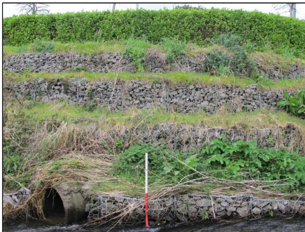
Plate 99: East-facing view of the four-tiers of stone-filled gabions used to delineate the river channel (1m scale).
