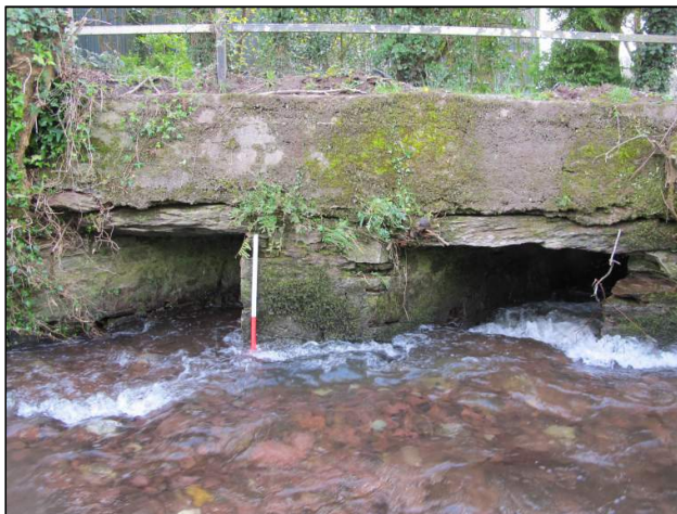
Plate 147: South-facing view of angled cutwater on upstream side of bridge, Feature F07 (1m scale).
