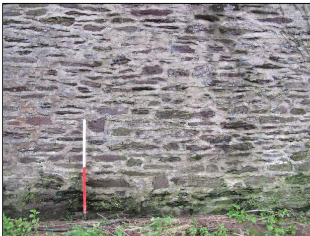
Plate 126: Example shot of masonry forming the arch-walls (east side of Arch No. 4) from Kilnap Bridge (1m scale).
