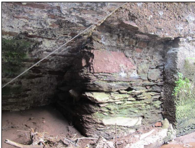
Plate 174: Stone wall and overlying concrete abutting the west side of the arch-ring from Feature F16.
