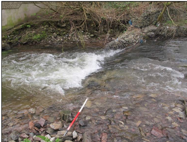
Plate 104: West-facing view of small weir that crosses the river-channel (1m scale); see Figures 17 for location.
