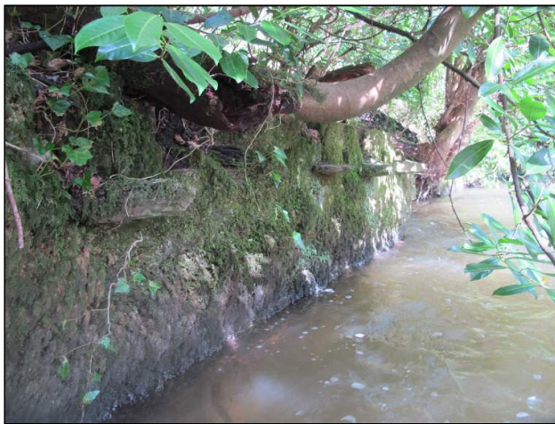
Plate 141: North-facing view along bonded masonry wall section (Feature F04B) located on the west side of the river.
