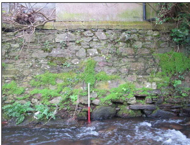
Plate 156: Detail shot of river-walling (Feature F10); note drain feature to bottom right of picture (1m scale).
