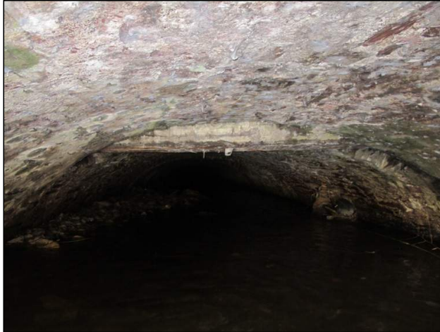
Plate 175: Internal shot of Intrados from section of culvert, Feature F16.
