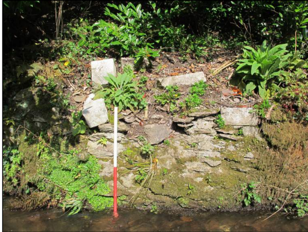
Plate 142: Section of bonded masonry walling that accommodated a footbridge across the river channel (1m scale).
