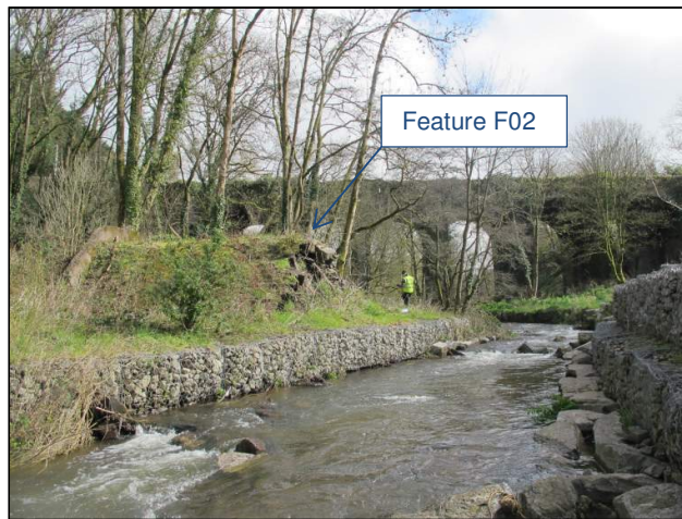
Plate 128: View of Glenamought River between Kilnap Bridge and Kilnap Viaduct; note remains of Feature F02 (Weir/ Dam structure) situated on west side of the river channel.
