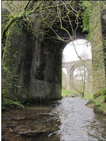
Plate 124: Southwest-facing view of Glenamought River flowing through the fourth arch of Kilnap Bridge (Feature F01); note Kilnap Viaduct (Feature F03) in distance.
