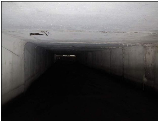
Plate 116: Internal view of culvert showing box-section concrete used in its construction.
