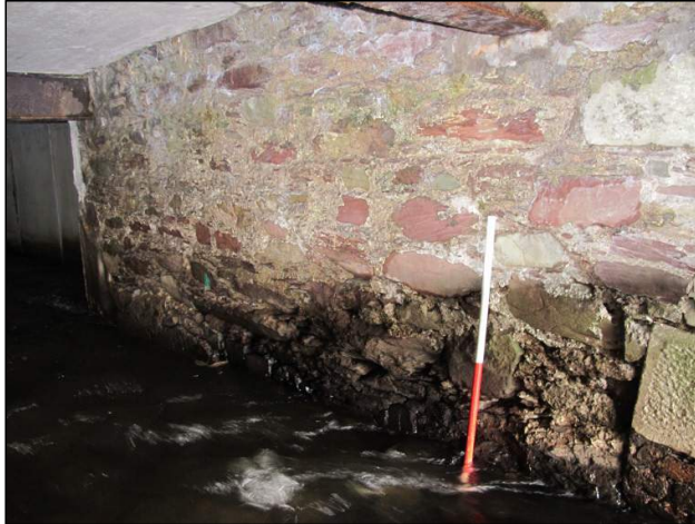
Plate 163: Masonry wall that extends southward from culvert arch, Feature F12 (1m scale).
