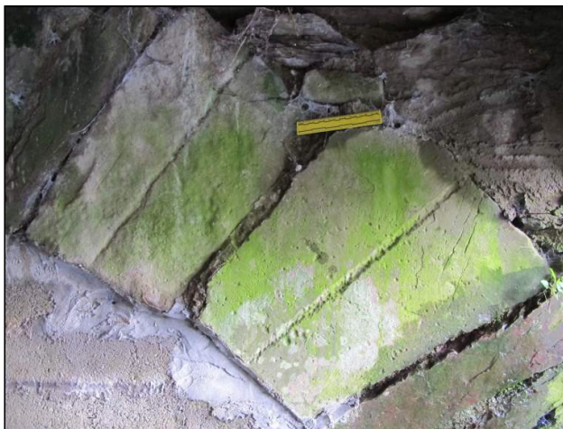
Plate 162: Detail shot of limestone voussoirs (S2 and S3) which have punch lines running down their centre (15cm).
