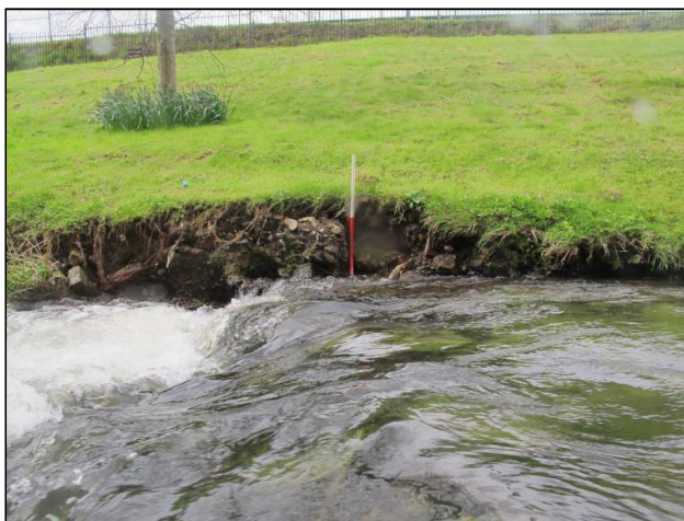
Plate 96: Line of boulders forming a small weir that extends across the channel (1m scale); see Figures 16 for location.
