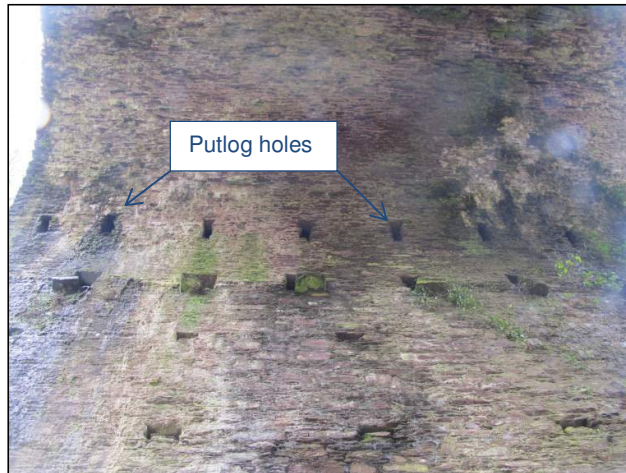
Plate 127: View of top of arch-wall and east side of the intrados from Arch no. 4; note the presence of a series of putlog holes.
