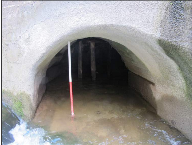
Plate 118: Culvert that drains into the river on its east side, upstream of the Watercourse Road Culvert (1m scale); see Figure 18 for location.
