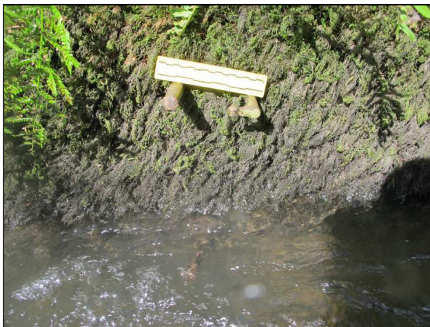
Plate 138: Wrought-iron fastenings protruding from river walling, Feature F04A (15cm scale).
