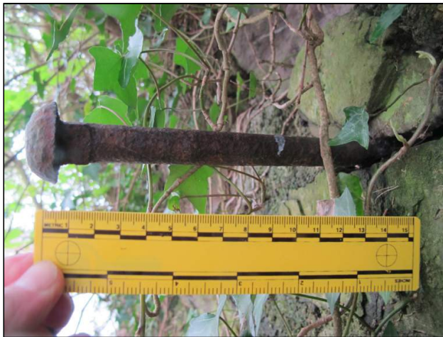
Plate 158: Round-headed iron pin protruding from river-walling, Feature F10 (15cm scale).
