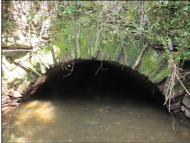
Plate 166: North-facing view of the downstream arch-ring from masonry culvert running beneath watercourse road (Feature 14A); see Figure 19 for location.
