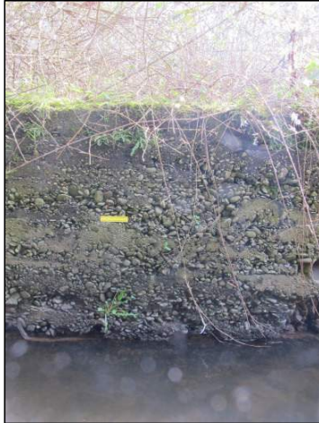
Plate 121: East-facing view of section of modern river-walling located along a c. 63m section of the watercourse, on its eastern side (15cm scale).
