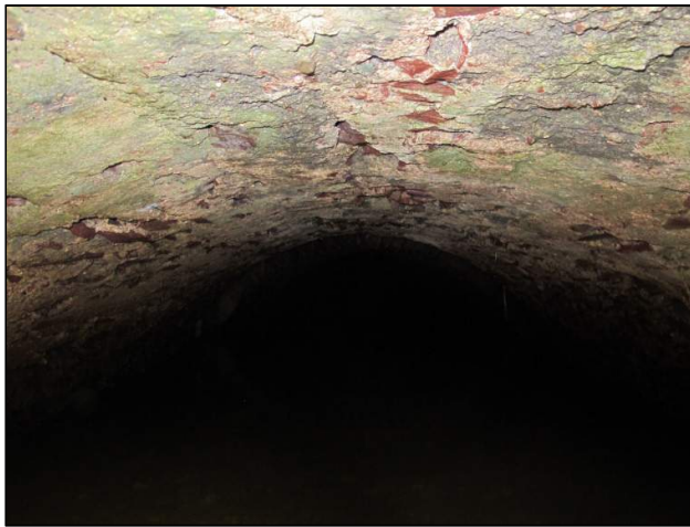
Plate 167: Internal shot of Intrados from section of culvert, Feature F14A.
