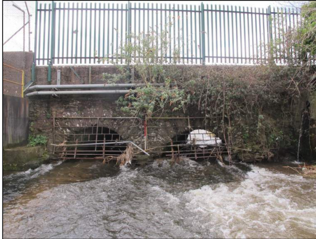
Plate 151: Northwest-facing view of downstream side of masonry bridge (Feature F09) at Fitz's Boreen (1m scale).
