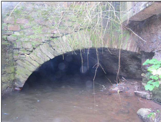
Plate 173: South-facing view of arch-ring forming entrance to culvert, Feature F16; see Figure 19 for location.
