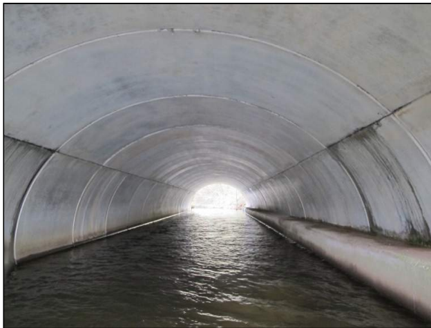
Plate 101: Internal view of modern culvert that accommodates river-flow beneath the N20 roadway (1m scale).
