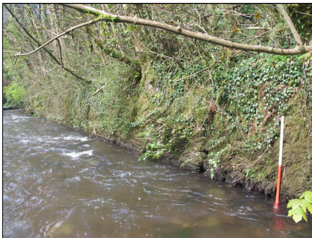
Plate 135: Southwest-facing view of section of river-walling (Feature F04A) that delineates a 78m section of the Glenamought River on its north side (1m scale).
