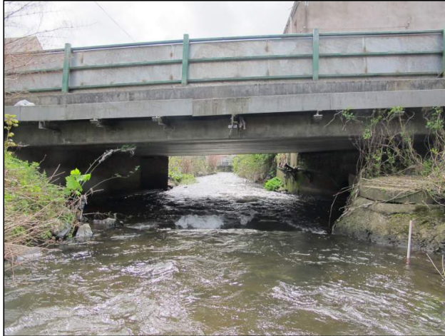
Plate 112: South-facing view of upstream side of modern culvert that provides pedestrian access to Orchard court from the Commons Road (1m scale).
