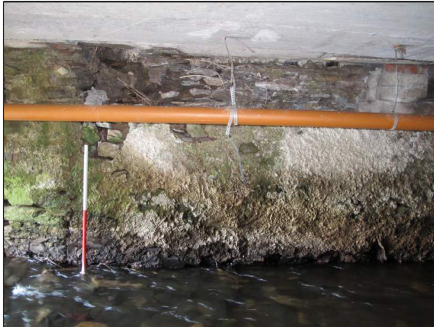
Plate 164: Masonry wall comprising the east wall of the main culvert, located opposite Feature F12 (1m scale).
