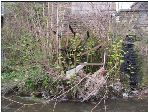
Plate 111: Shot of disused water-wheel located on west side of the river channel (1m scale); see Figure 17 for location.
