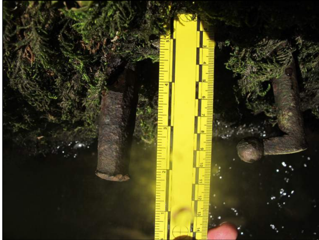
Plate 139: Wrought-iron fastenings protruding from river walling, Feature F04A (15cm scale).
