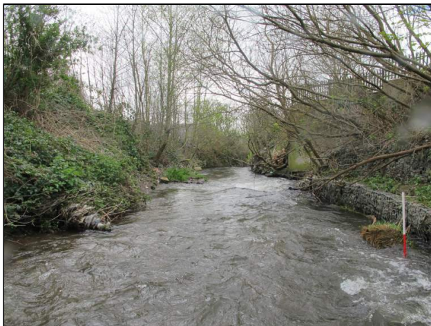
Plate 102: South-facing view of River Bride on downstream side of culvert, north of Vaudeville Terrace (1m scale).
