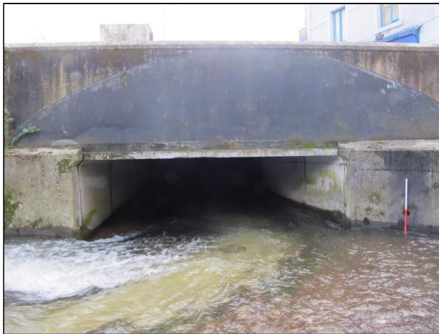
Plate 119: Upstream side of modern culvert that forms the northern side of the culvert running beneath Watercourse Road (1m scale).
