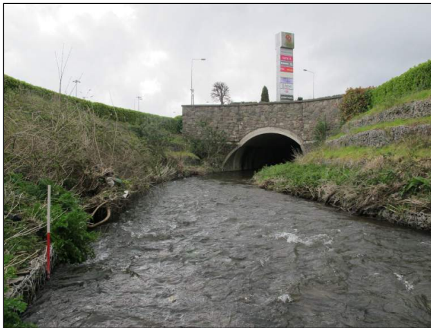
Plate 98: North-facing view of river channel on downstream side of culvert/ road bridge, note stone-filled gabions used to form the attendant banks (1m scale).
