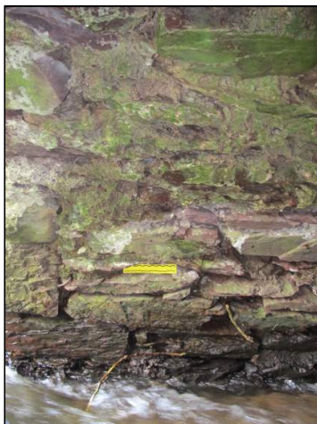
Plate 153: Example shot of masonry forming arch walls of Feature F09 (15cm scale).
