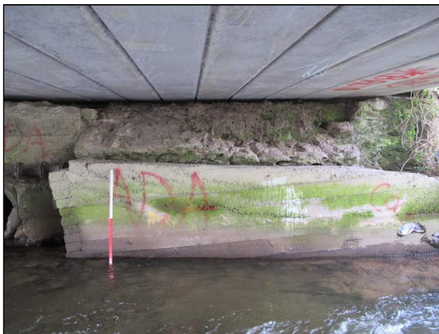
Plate 159: West-facing view of remains of masonry bridge (Feature F11) located beneath modern culvert at Orchard Court (1m scale); see Figure 18 for location.
