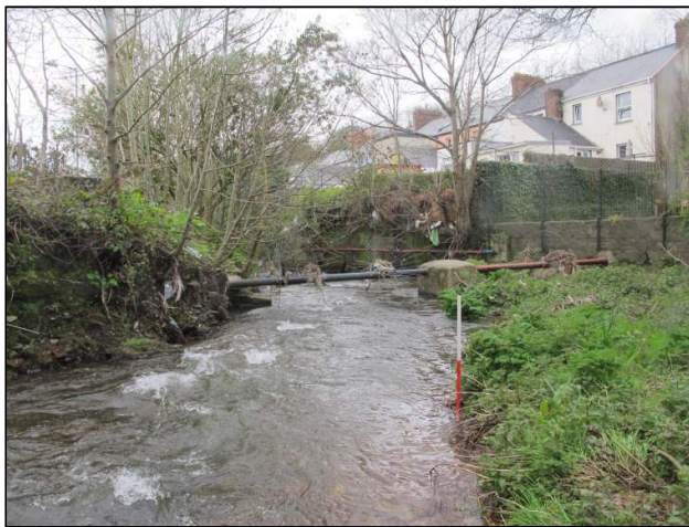
Plate 105: Iron-pipe that crosses the river, immediately upstream of Vaudeville Terrace (1m scale); see Figure 17 for location.
