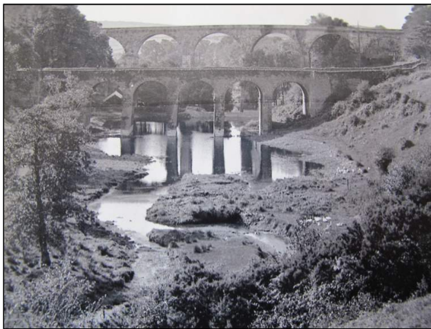
Plate 132: Early twentieth-century photograph showing millpond/ lake created by the presence of a dam structure (Feature F02) located upstream of Kilnap Viaduct [Photo courtesy of owners of Kilnap Glen House].
